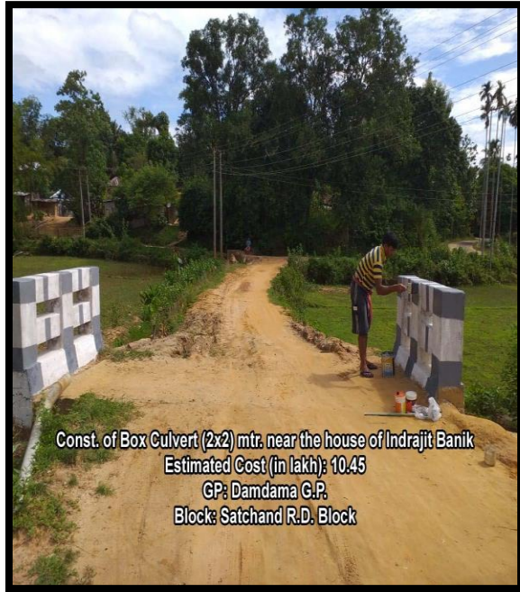
Name of Work: RCC Box Culvert GP: Damdama Block: Satchand District: South Tripura
