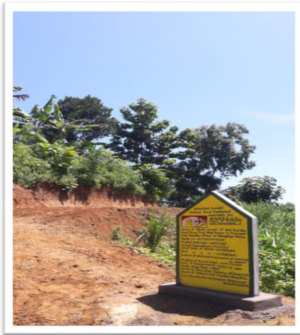
Name of Work: Formation of Road GP: Ailmara VC Block: Shilachari District: Gomati
