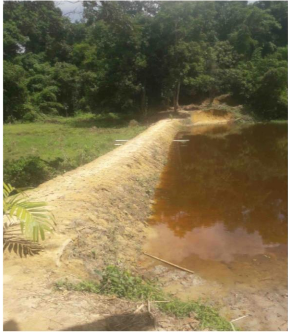
Name of Work: Earthen Check Dam GP: Dhanlekha VC, Block: Ompi District: Gomati
